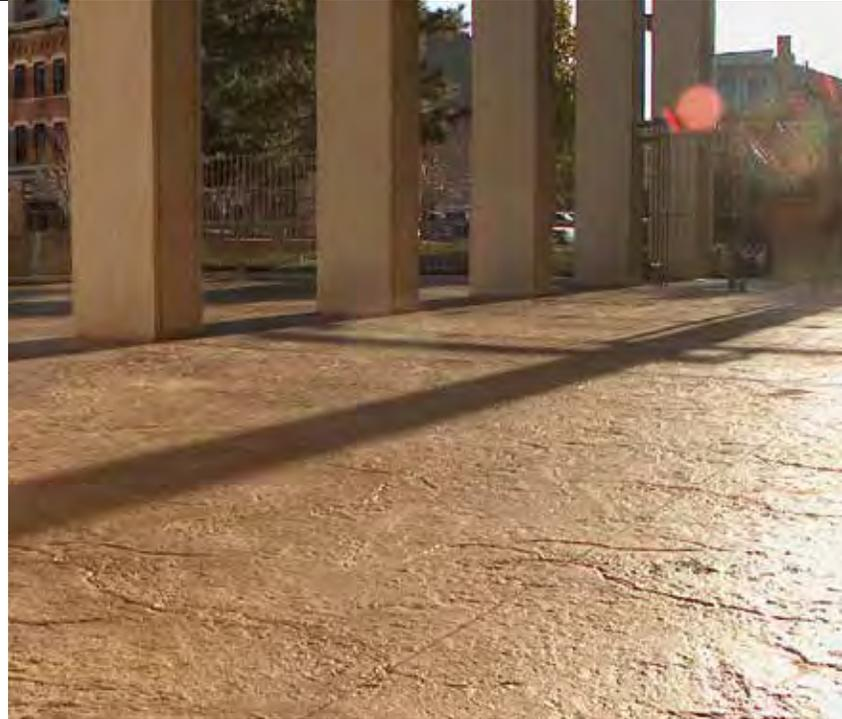
Brickform Stampable Overlay "Gray" is a premixed blend of special materials that, when mixed with water, forms a thin, concrete coating. This overlay is intended for use with Color Hardener and Antique Release.
